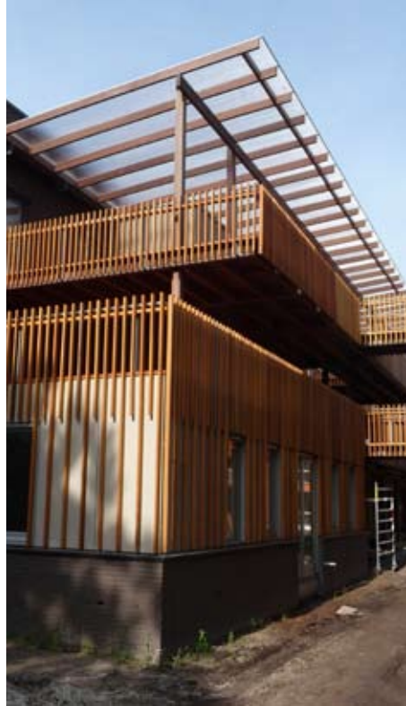
Guariuba (Clarisia racemosa) in new construction building Erica (photo: Wijma Kampen B.V.)
