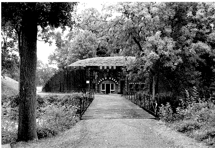
Extensive vegetation at Fort Rijnauwen today (Photo: Titia Blom. See also colour page 25)
