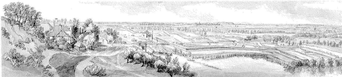
View from the Heimenberg of the hamlet of Grebbe and the hornwork on the Grebbe dam (17 July 1750, Jan de Beijer. Het Rondeel Museum Civic Collection, Rhenen). In this drawing, made some years after the construction of the hornwork, planting is yet to be seen.
